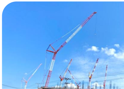
Torch Tower 建設工事 (HVO100%)
